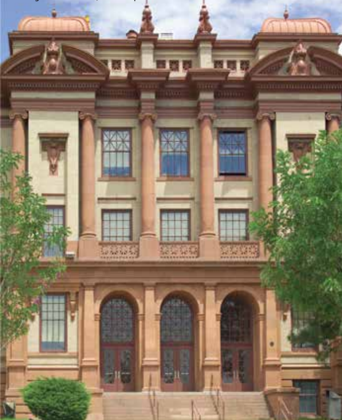
North High School, Denver, CO Humphries Poli Architects
